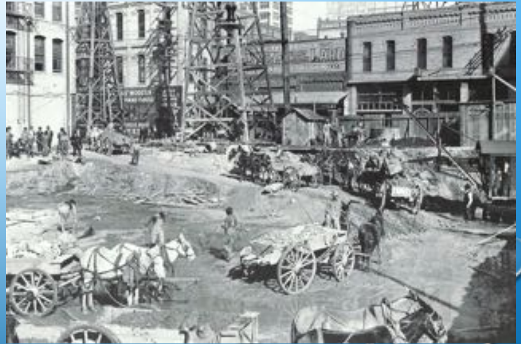
Artesian well being drilled at Adolphus Hotel, Dallas, Texas Source: www.youhavewatermail.blogspot.com
